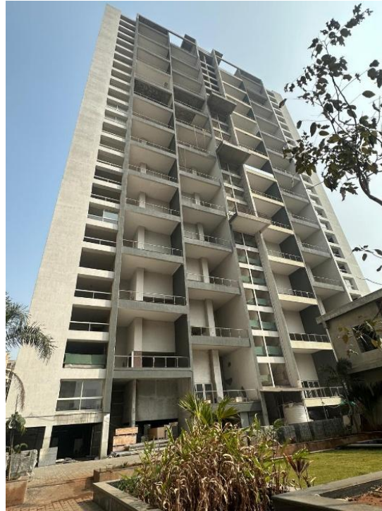
Fig A – Site Photographs
